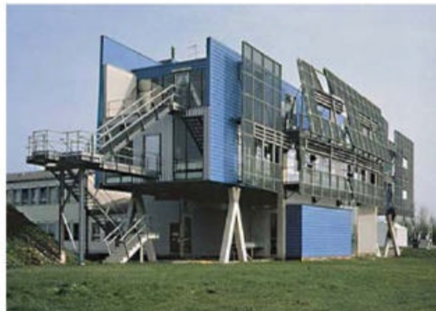
Office and Research Center Seibersdorf, Austria 1995
